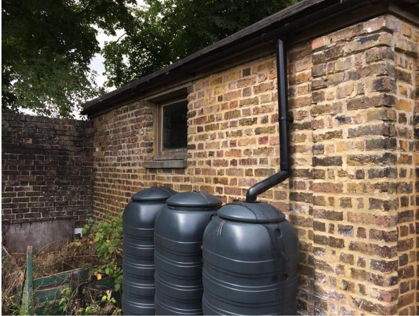
With your butts in place and properly connected, you can start harvesting rainwater. Once you have a substantial quantity of water stored you can reap the rewards. Even with a small shed, you can start the season with two full water butts, enough to fill up 50 watering cans. During the summer your water butts will get a regular top up. That means fewer trips to the pump, and the ability to fill your watering can just by turning on the tap.
